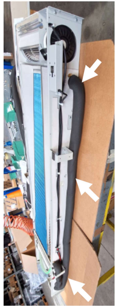
PUT INSULATION IN ALL THE EXTERNAL PIPE
